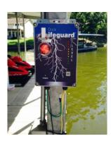
• Metal Floating Docks unbonded to a Common Ground that carries Voltage: Some lake environments are such that the Common Ground carries Voltage on it. Because of this, the dock may be wired in PVC Conduit, and not bonded to the dock frame to avoid providing a path for this voltage to get onto the dock frame and into the water. The green Ground Reference Wire should be mounted to the dock frame.
