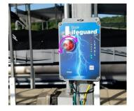
• **Alarm Volume**: Volume of the siren can be adjusted by twisting the clear ring that on the outside of the red alarm light.
