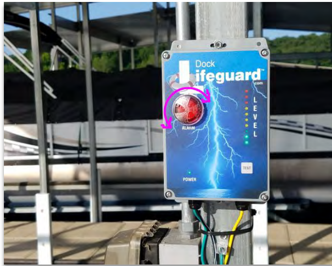
Figure 6, Rotate Clear Ring Over Red Light to change Volume Level
